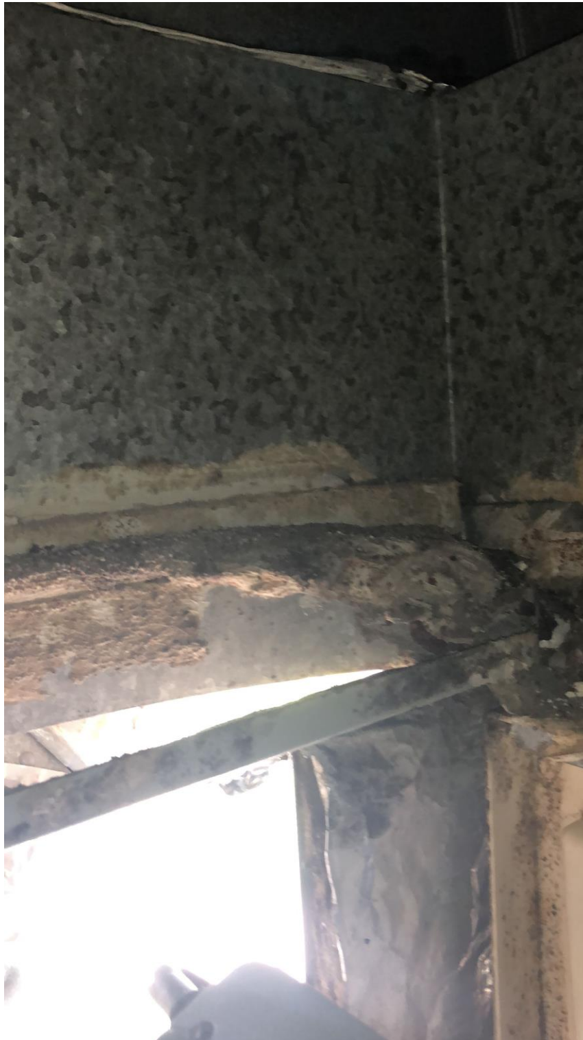
Mold in HVAC unit two months AFTER November 2018 remediation (Laughlin AFB)
