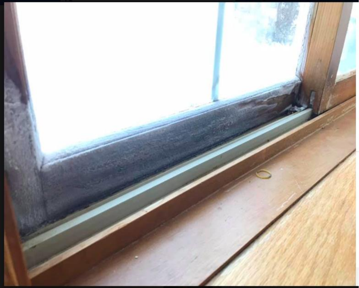
Mold on the Window ( Minot AFB )
