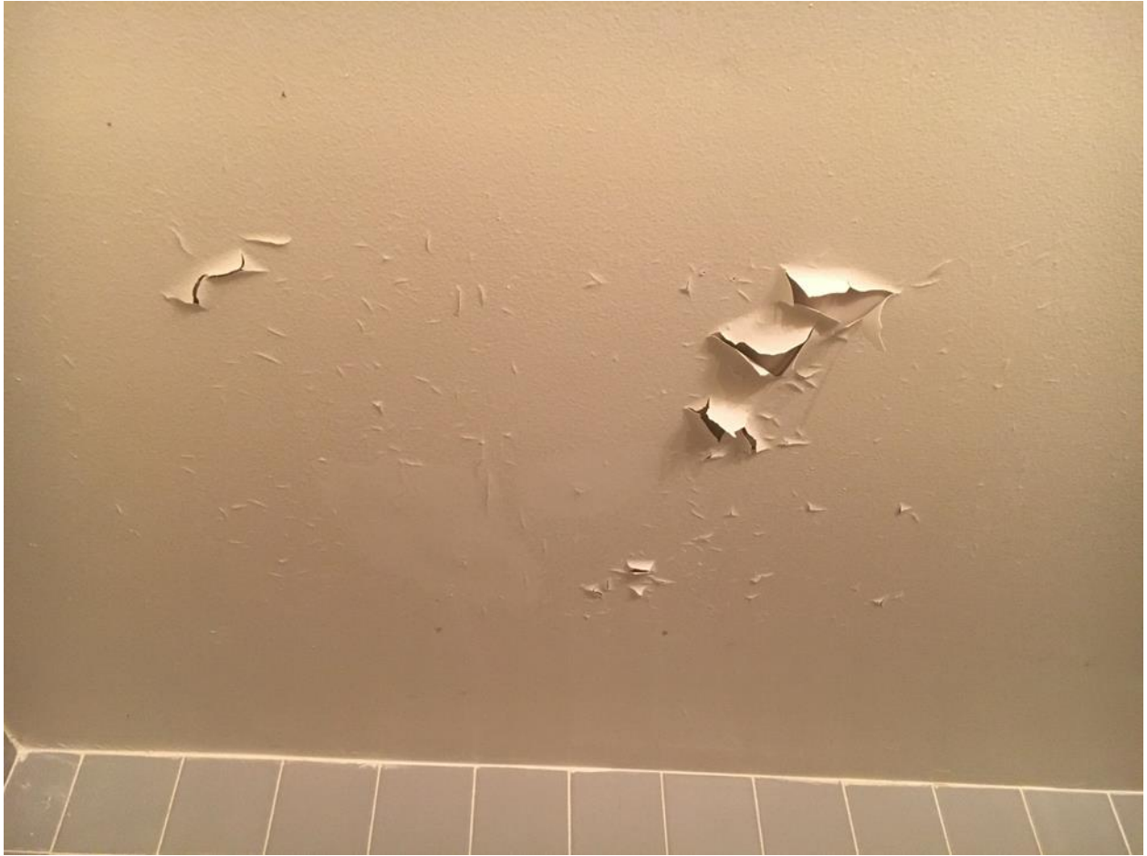
Chipping paint falling off the walls and ceiling (MCAS Beaufort)
