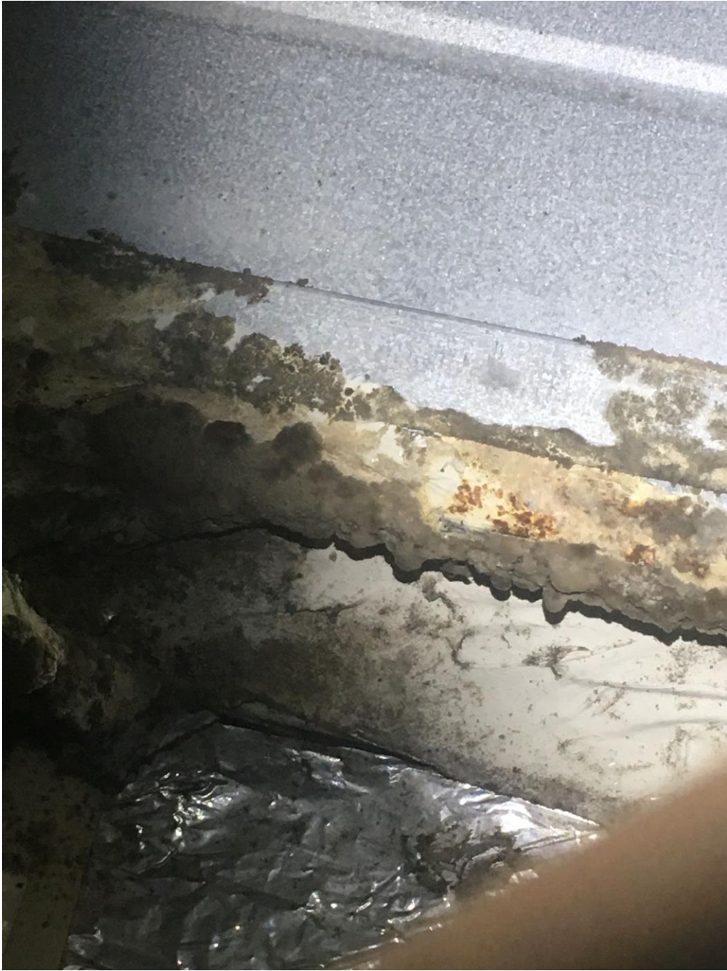
Mold in HVAC unit prior to November 2018 remediation (Laughlin AFB)
