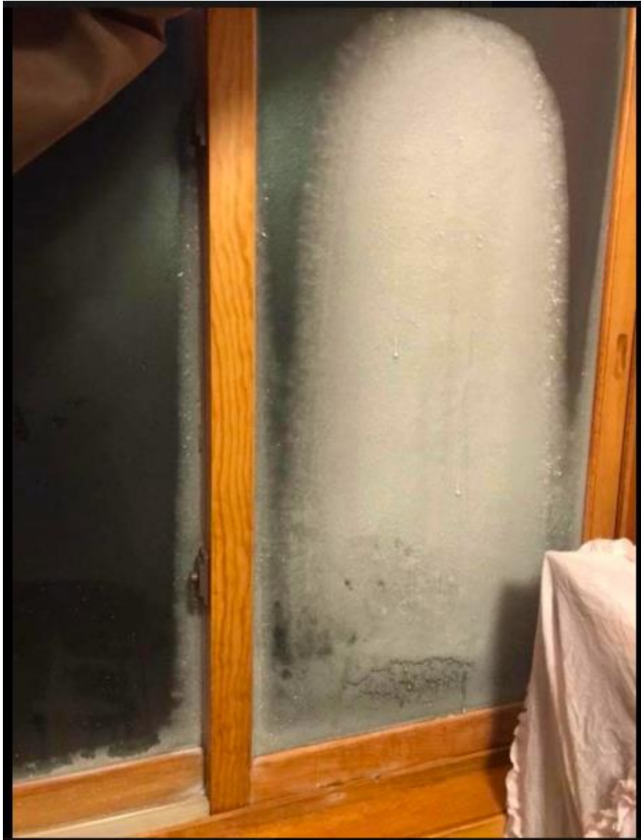
Frost and Ice inside the Window (Minot AFB)
