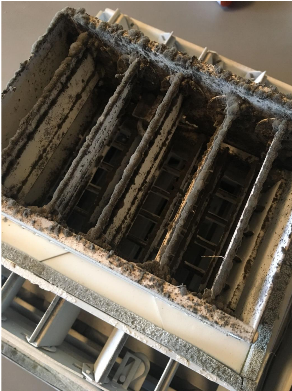
Mold on air registers prior to November 2018 remediation (Laughlin AFB)
